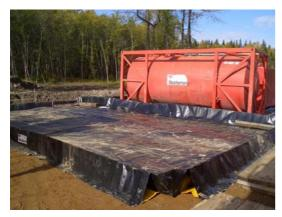
Figure 18: Part of environmental measures, bunding used to isolate water supply for hydrotesting
