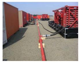
Figure 17: Bunding for any diesel driven equipment was extensive
