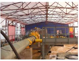
Figure 13: Above ground pipeline section protected by habitat
