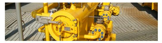
The locking system prevents the operator from operating a valve when it is not allowed and the valve can only be operated with the designated key. Each lock is operated by two keys, one released in the open position and one in the closed position. By using unique keys that travel between locks the key codes can be designed to guarantee the steps of operation and guide the operator through the sequence.
