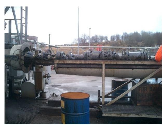
Receipt of not clean 16" Ultrasound- based ILI after un-successful inspection of TOR1 pipeline at Mongstad 2006
