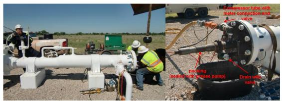
Figure 13: Tool loading (left) / launcher set-up (right)
