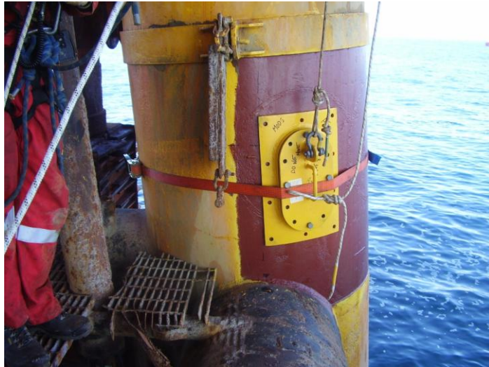
Figure 3: The access for a keyhole inspection of a leg
