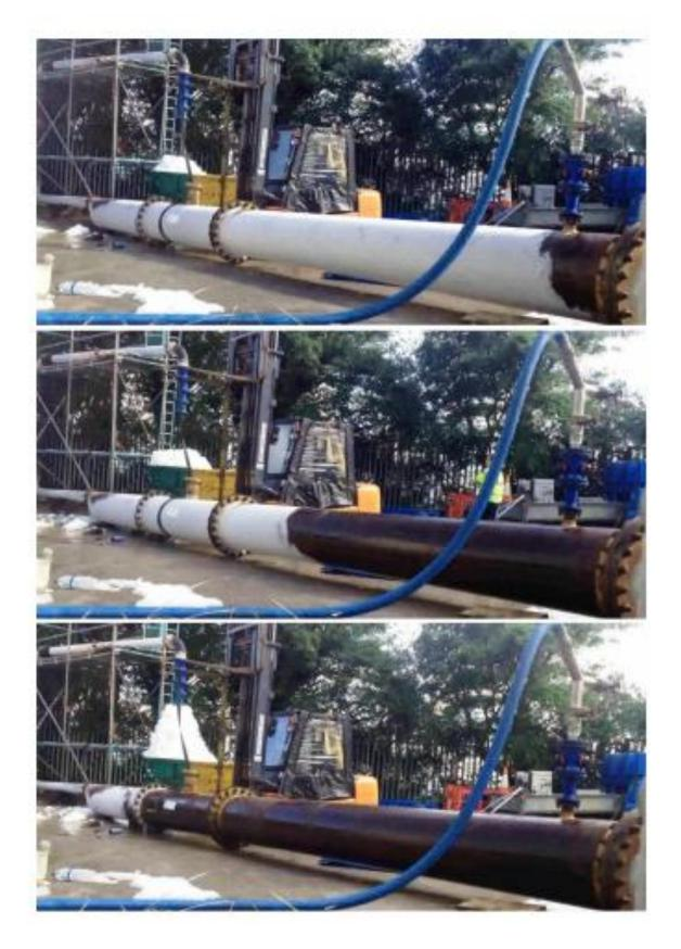
Figure 3 Ice pigging was performed on a dual diameter 24" to 8" steel pipe. The ice and push-water were inserted through a 2  $\frac{1}{2}$ " hose connected to a 2" inlet. Frozen condensation on the pipe shows the progress of the ice plug through the constriction.
