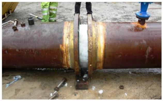
Figure 5 A compressed ice pig holds its shape as the pipe is opened up for inspection.
