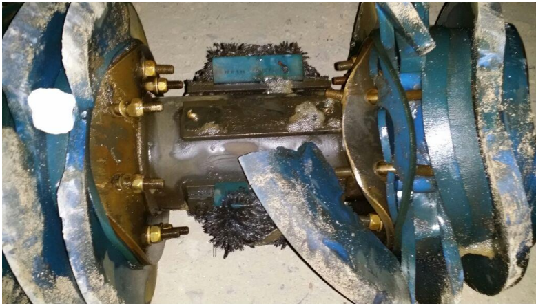
Scraper Damage During Pre-Comm
