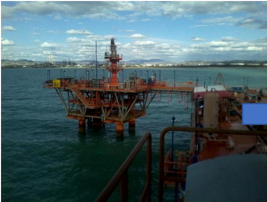
Requires ILI Inspection but Pipeline has no run history
