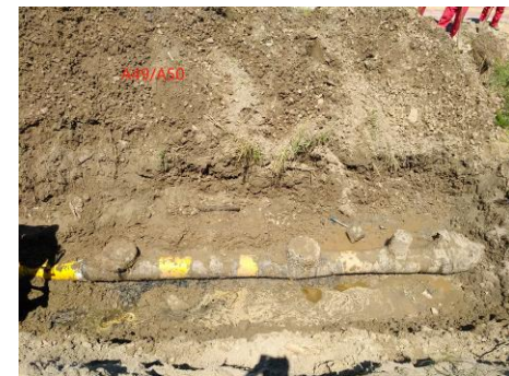
Pipe Excavated & Hot Taps Identified
