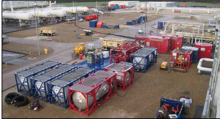
Figure 6: 36-in., 118.7-km Gas export pipeline onshore flushing station
