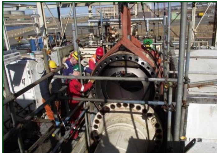
PLR Isolation Valve, In-Situ Repair
