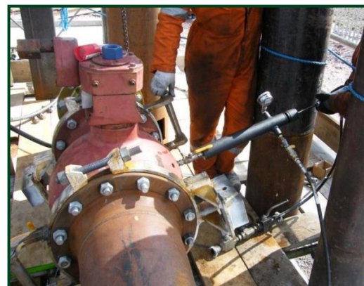
4. Fit valve and small-bore hot tap machine to the tapped connection – leak test entire assembly
