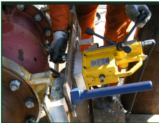
1. Drill initial hole to specified depth
