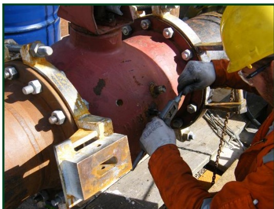
3. Manually tap to cut the thread into the hole
