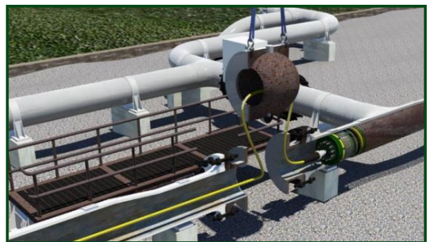
In-Situ Repair Using a Tethered DBB Tecno Plug - Production Unaffected
