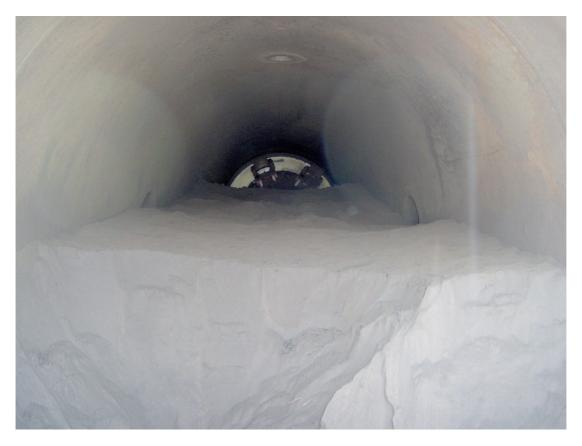
Figure 3: Receiver filled with black powder
