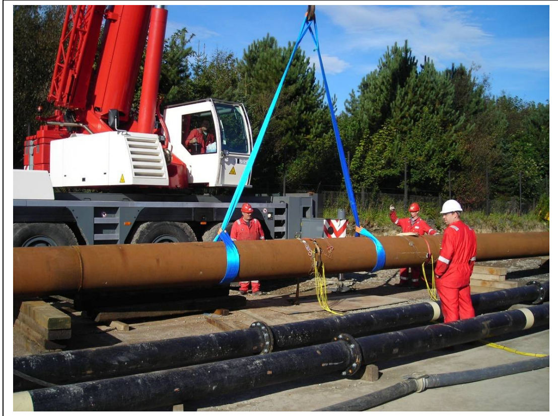
Figure 7 - Bending the Pipe
